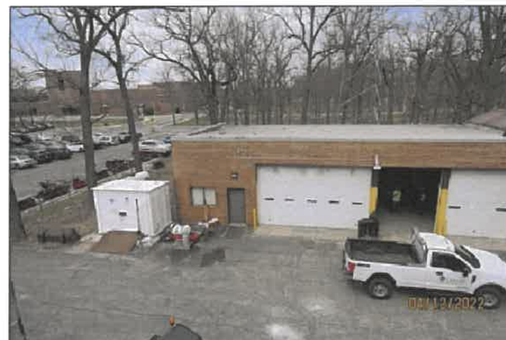
LOW SLOPE ROOF - VIEW 2
