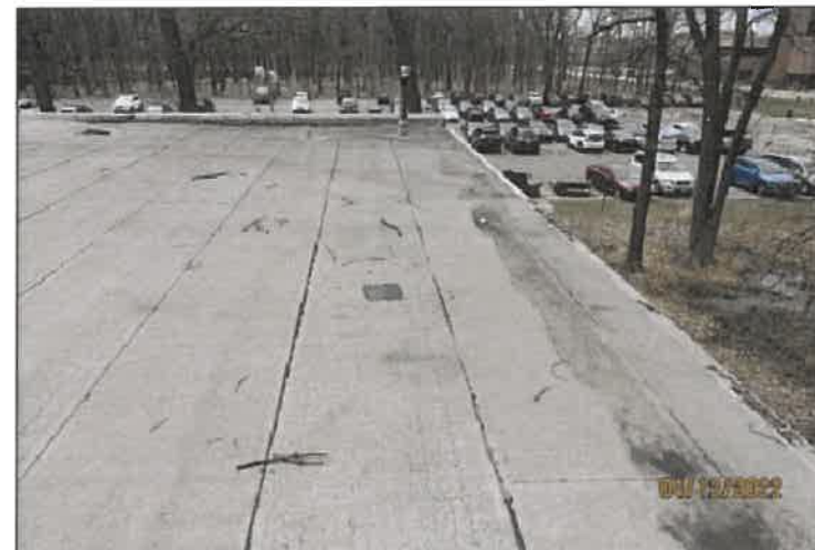
LOW SLOPE ROOF- VIEW 1
